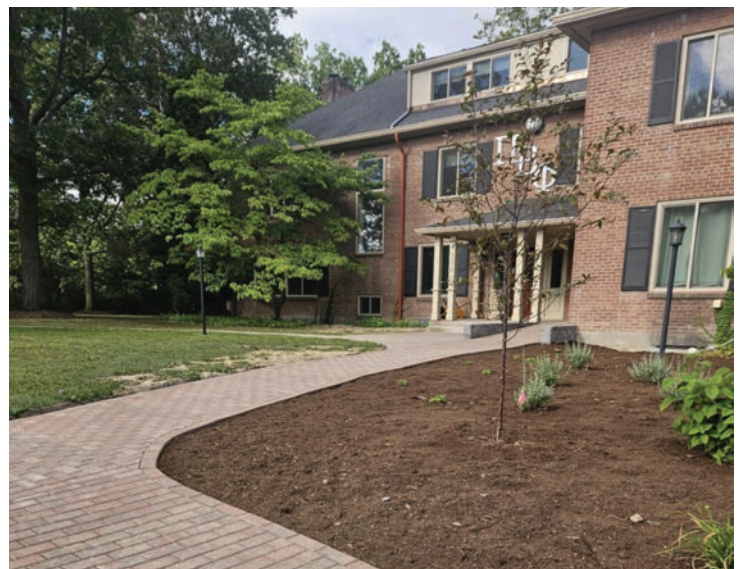
After with front sloped sidewalk.
