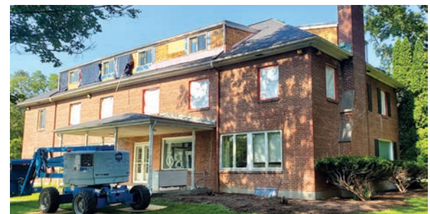
Windows being installed on the second and third floors.
